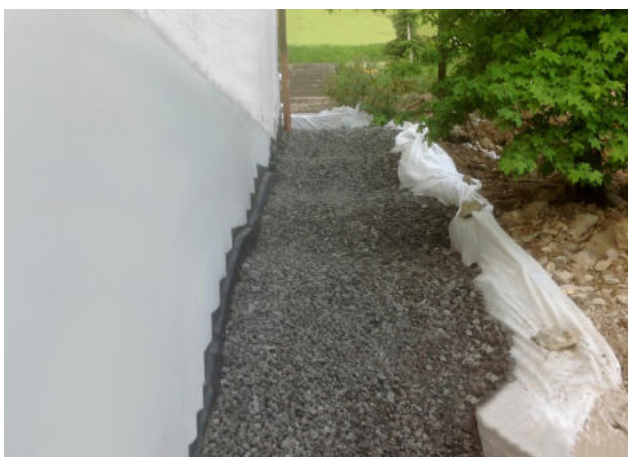
Filling in the working pit and compressing GEOMATERIALS Foam Glass in layers
