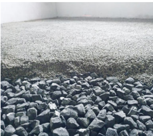
Foam glass aggregate cement-bounded, Yard Mittergroßbefehn, Germany
